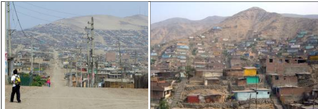
Figure 1: Nueva Pachacútec and Húascar, suburbs of Lima without water supply and installation of some "dry sanitation systems" (dehydrating toilet with sand filter for urine and greywater)
